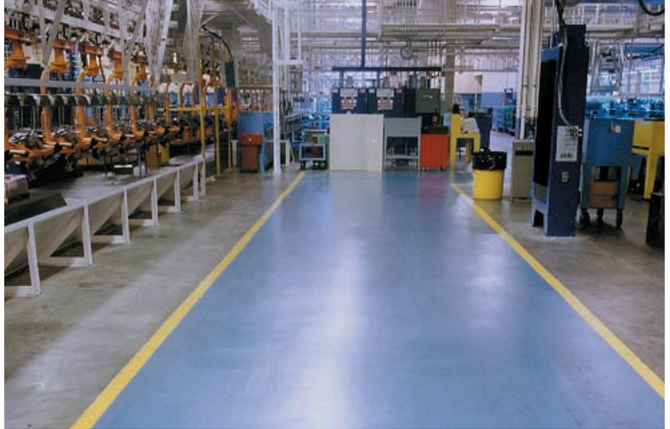
*Traffic aisle overlayed with Stonhard's Stonclad PT high-performance polymer flooring system provides a monolithic surface that's easy to clean and maintain. And, with an optional texture, provides a high level of slip-resistance for employee safety.*
