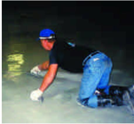
*After Coca-Cola's old epoxy mortar floor system was removed with jack hammers, the exposed concrete substrate was mechanically prepared. After preparation, Stonhard's specially trained installation team screed applied a four-component urethane mortar with quartz aggregate broadcast for texture. This was followed with a high performance urethane sealer for an extra measure of chemical and abrasion resistance.*
