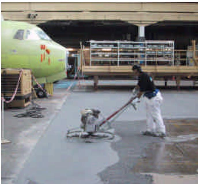
The final phase of the project involved creating discernible traffic aisles throughout the facility by applying Stonkote GS4 in bright white lines. The striped traffic aisles were easy to recognize and adhered to safety regulations ensuring a sound work environment.
