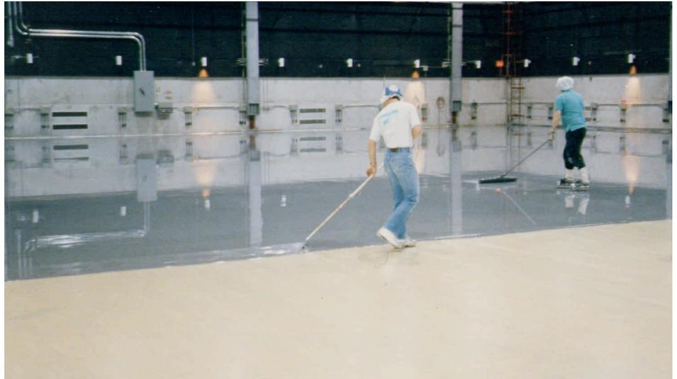
*Part Two: A second primer layer follows the first to provide conductivity and an additional seal.*
