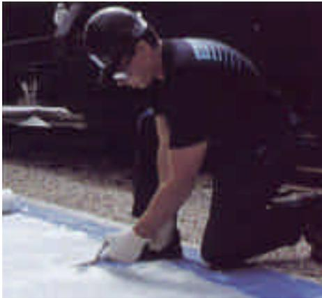
*Fiberglass engineering fabric is used in conjunction with epoxy membrane to isolate cracks in substrate.*
