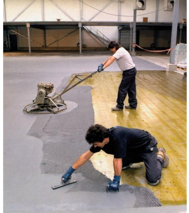
*A power trowel is used in wide open areas to produce a smooth, flat surface. The floor is attractive, easy to maintain, and makes it easier to operate wheeled vehicles.*
